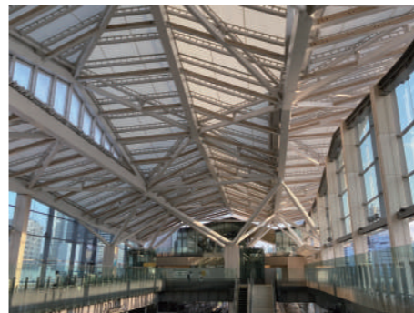
■ Takanawa Gateway Station Completed : 2020 Location: Tokyo
