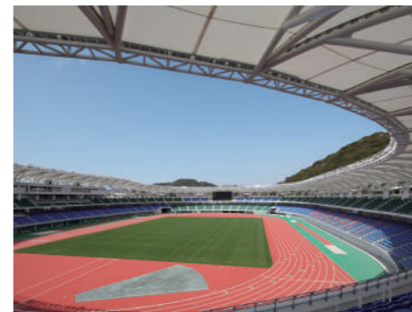
■ Nagasaki Prefectural Sport Stadium Completed : 2013 Location: Nagasaki
