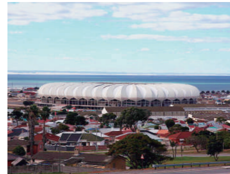
■ Nelson Mandela Bay Stadium Completed : 2007 Location: Republic of South Africa
