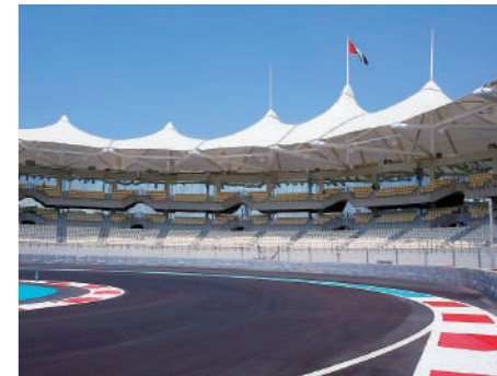
■ Yas Marina Circuit Completed : 2008 Location: Abu Dhabi
