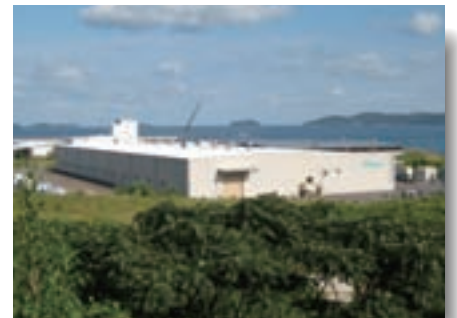
■ SC Plant (Manufacturing of silicon coating base materials) 851-46 Shimomen, Tsukinokawa-machi, Matsuura-city, Nagasaki-prefecture
